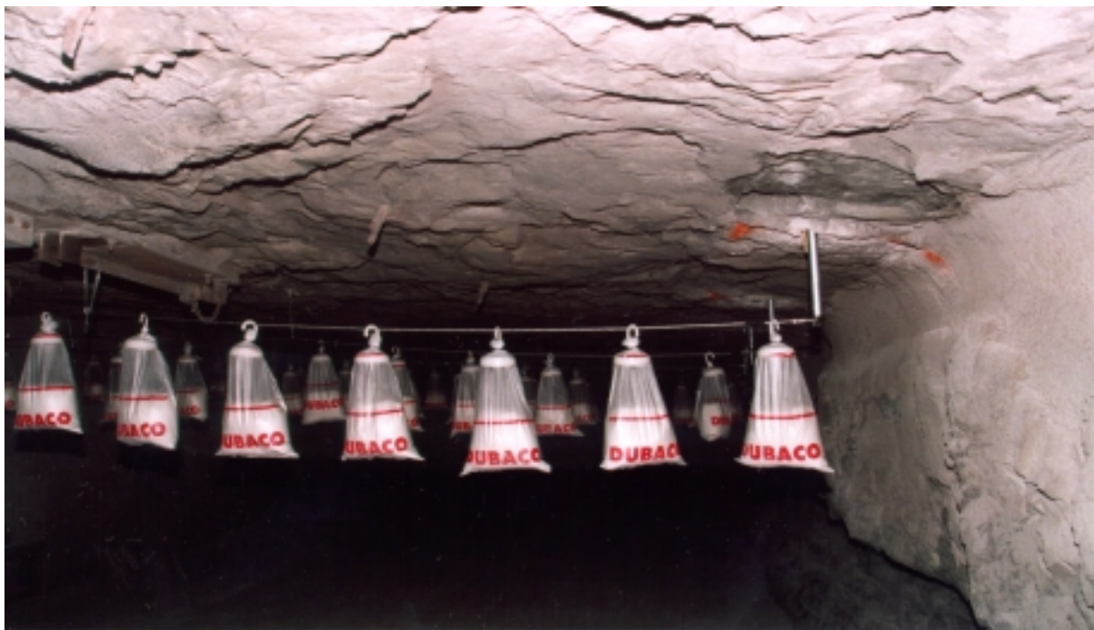
Figure 5.2.3b: Stone dust bags suspension method
